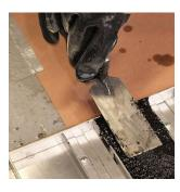
Initially smooth rough spots. Emcrete II is self-leveling and should not be "worked" too aggressively after it is poured into place.
