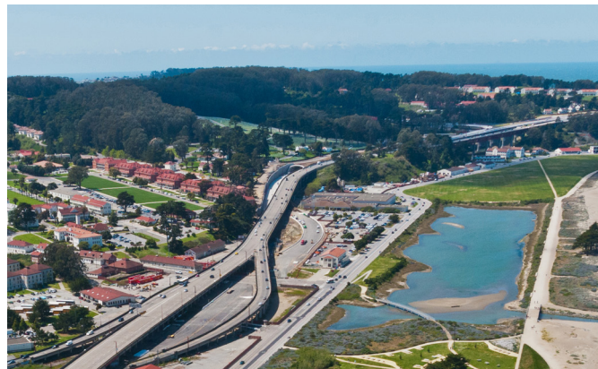
Presidio Parkway Viaduct San Francisco, CA
